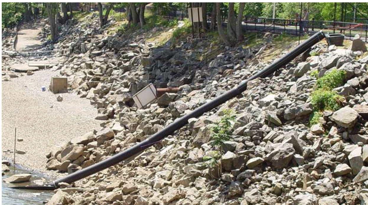
Figure 2. Experimental Eel passage pipe below Conowingo Dam, 2007
