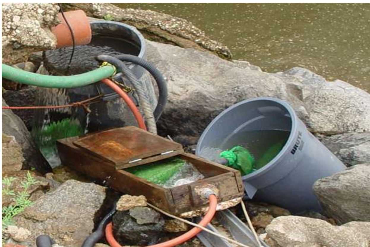
Figure 3. Irish elver ramp placed on rip rap in overflow from west fish left
