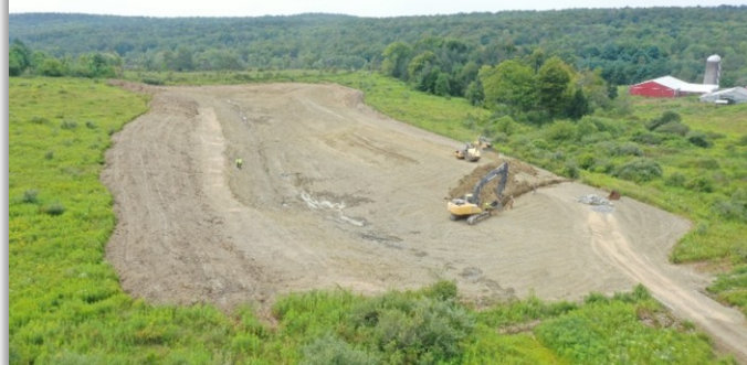
7-ft Basin during Construction of the Primary Outlet
