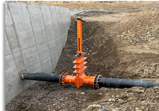
One of several safety valves in the system inserted into the welded gas line used to transfer the manure.
