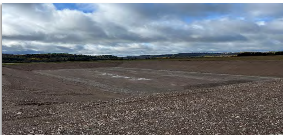
Site work complete with leak detection installed awaiting liner installation
