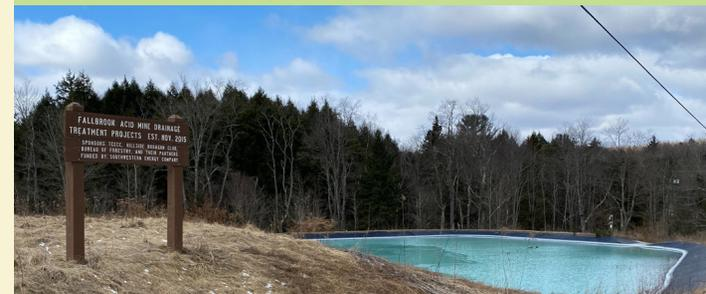
The Fall Brook facility uses three limestone beds and a polishing pond that remove toxic metals. The largely cleaned water is then released back into Fall Brook, a tributary of the Tioga River.
